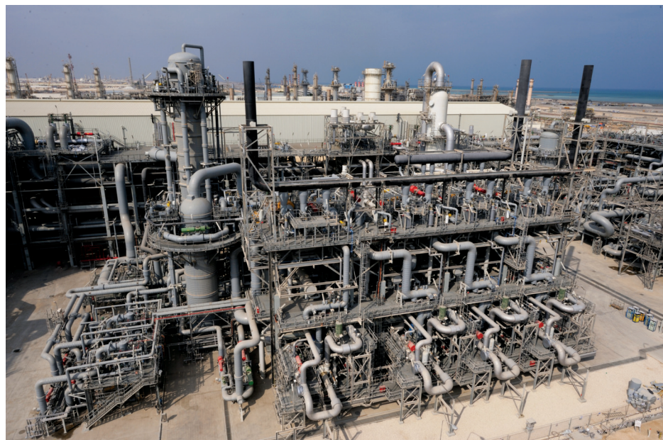
Air Products' AP-C3MR™ and AP-X® process technologies are in operation at the 14 existing LNG trains located in Ras Laffan, Qatar
